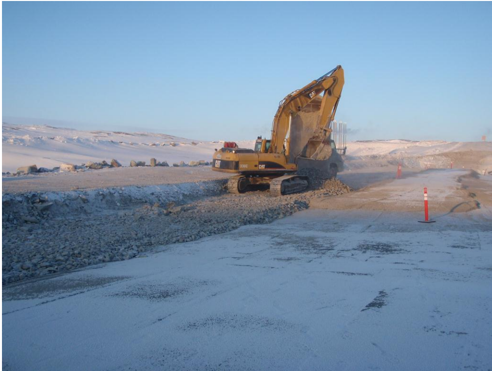
Photo 3: Excavator placing transition material along the downstream side of the dam.
