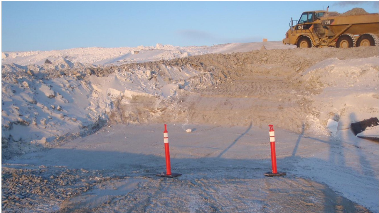
Photo 2: Removal of debris where the northern core ties in to original ground; this area will no longer be used as access.
